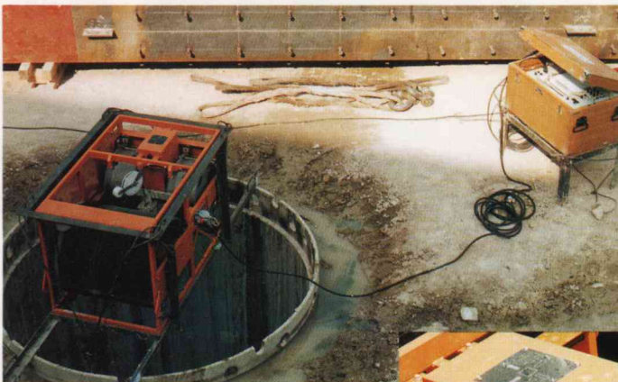
The winch unit located over a drilled hole.
